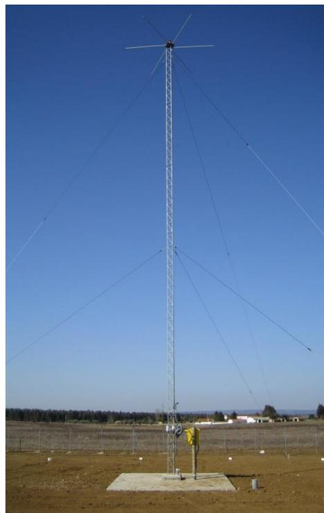
Figure: ground NDB installation
