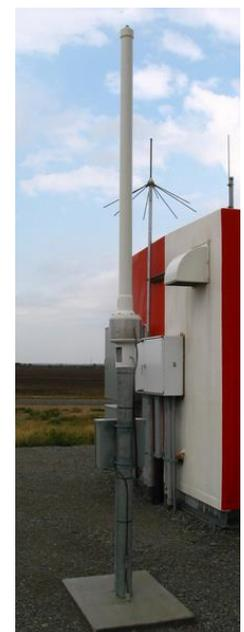
The distance measured by the aircraft is the direct path between the aircraft and the antenna of the DME. It is not the ground distance!
